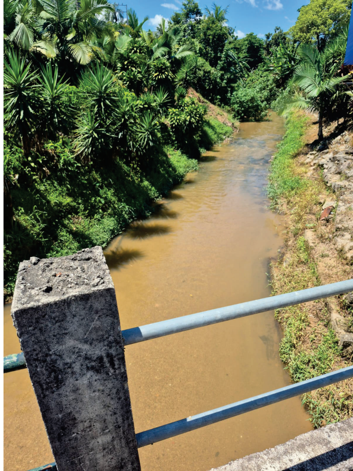
Figure 12 – Bridge 2 test site: 4.1 meters from guardrail to water surface.
