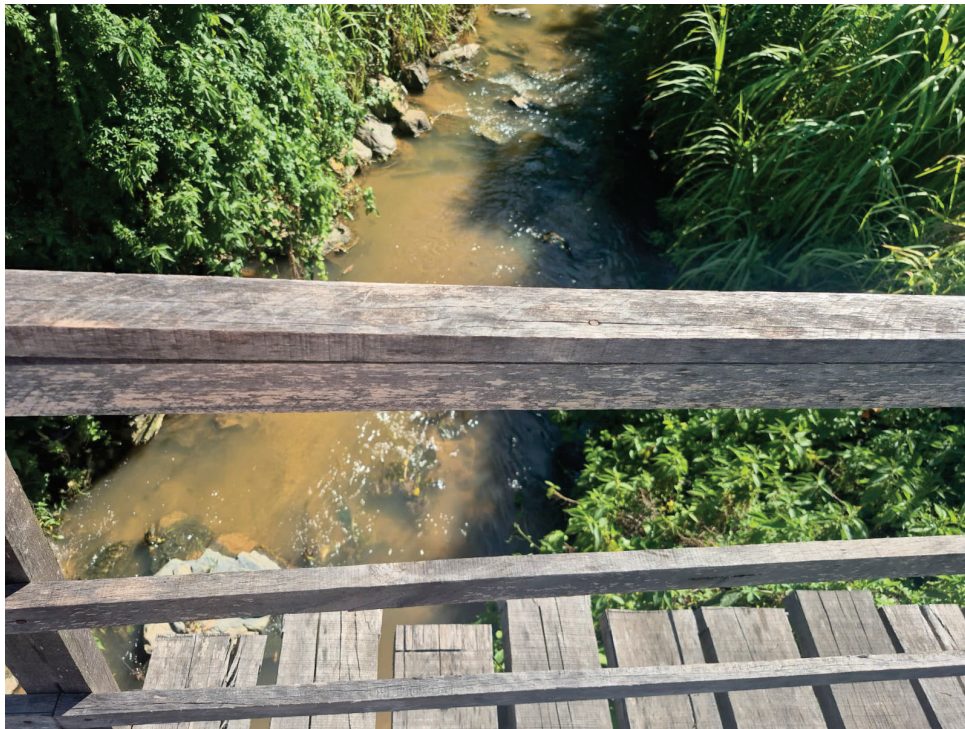
Figure 11 – Bridge 1 test site: 5.4 meters from guardrail to water surface.
