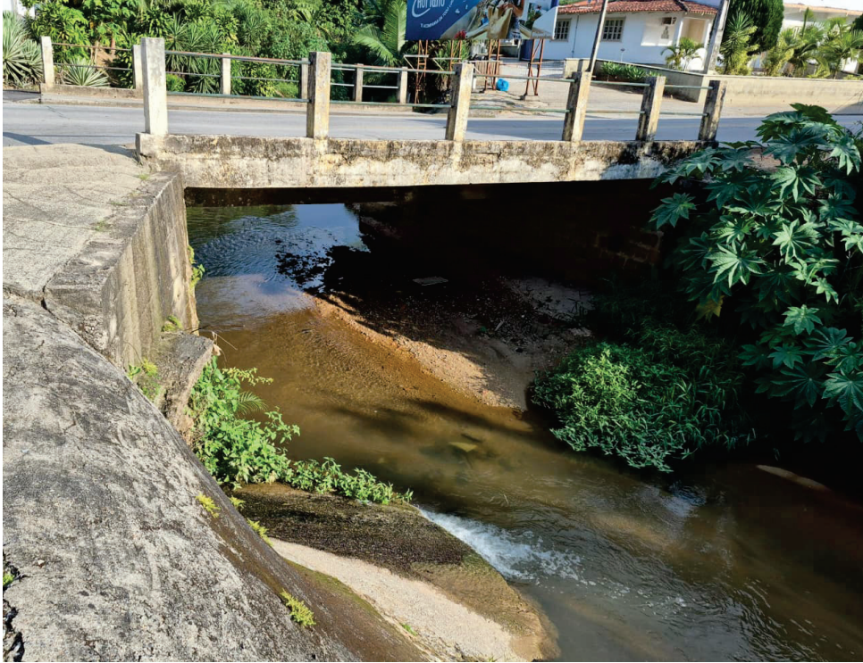
Figure 13 – Lateral view of Bridge 2 from the river margin, showing the bridge structure and surrounding environment.
